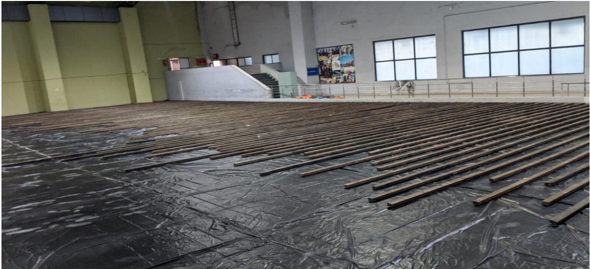
Installation of wooden flooring
